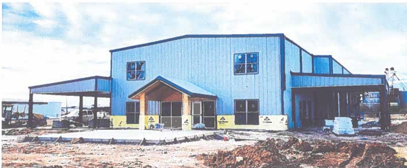
Briscoe Animal Resource Center, Uvalde – Under Construction
